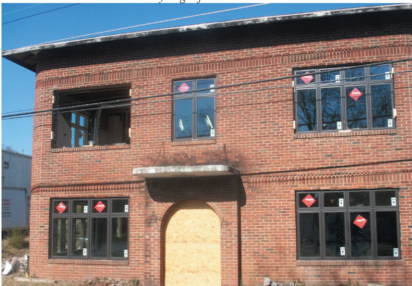
Early stage of the renovation.
