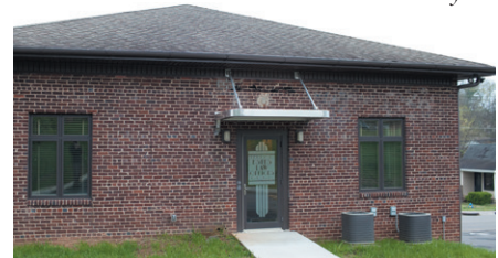
Estes opened a temporary office on Cook Drive while the restoration was underway.
